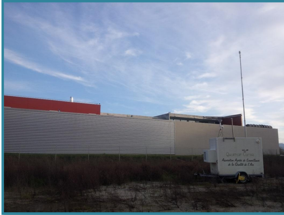
Figure 2 : Station mobile installée à la station d'épuration de Campo Dell'Oro (Source : Qualitair Corse).
